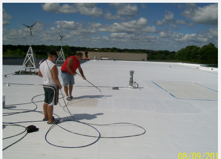
APPLY TWO COATS OF FINISH COATING
